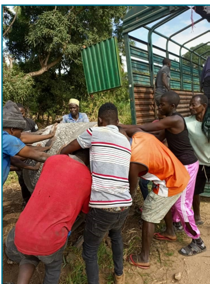
Unloading the well parts
