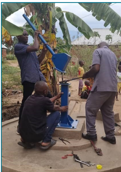
Installing the final pieces
