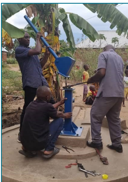
Installing the final pieces
